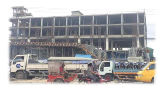
Collapse of concrete structures due to incorrect scaffolding installation and foundation preparation in construction site-one death and two injured.
