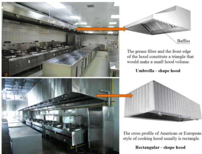
Fig. 2. The types of exhaust hood commonly used in the commercial kitchens.
