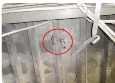
◁Inflicted damage on the floor and ceiling of ground floor due to the explosion▷
